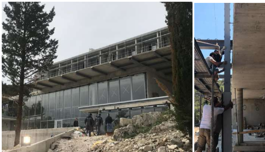
Figure 10 Glass facade of Hotel Osmine in Slano
