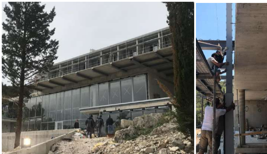
Figure 10 Glass facade of Hotel Osmine in Slano
